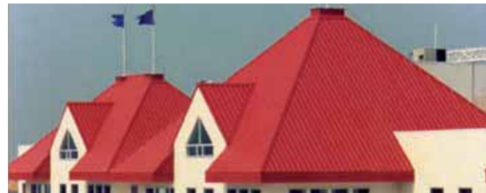
Above: Berridge R-Panel Roof
