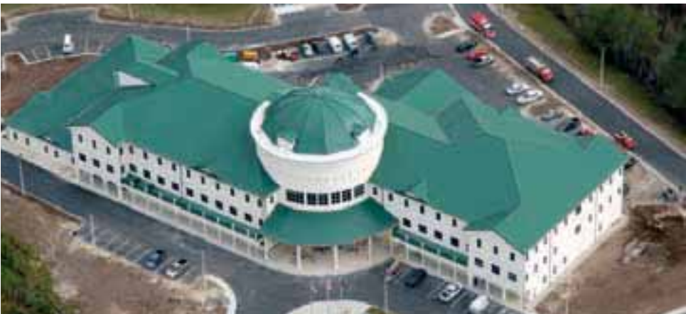
Above: Berridge Curved & Tapered Tee-Panel and Zee-Lock Standing Seam.
