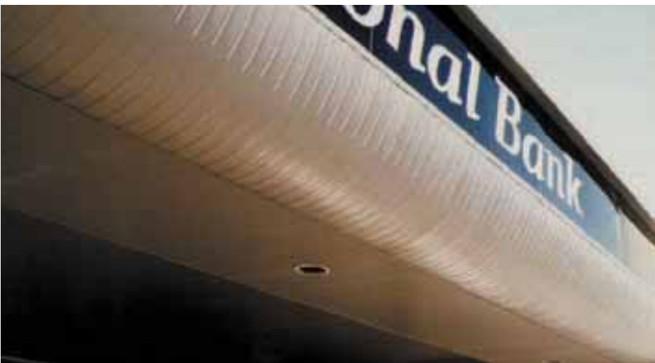
Above: Berridge Curved Flat Seam Panel
