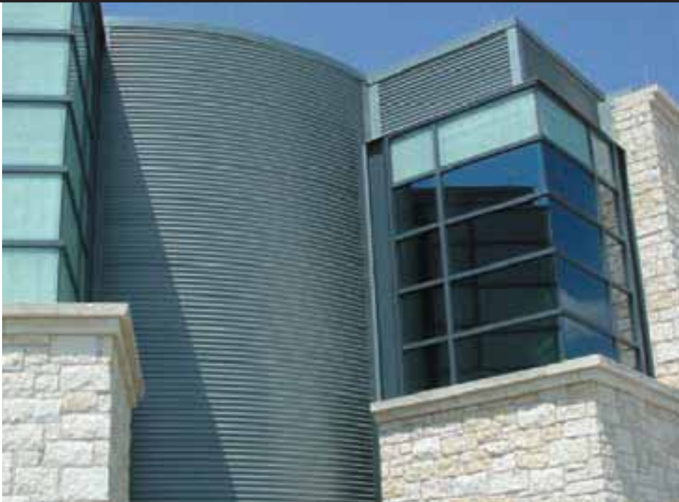
Above: Berridge Curved S-Deck - horizontal wall application
