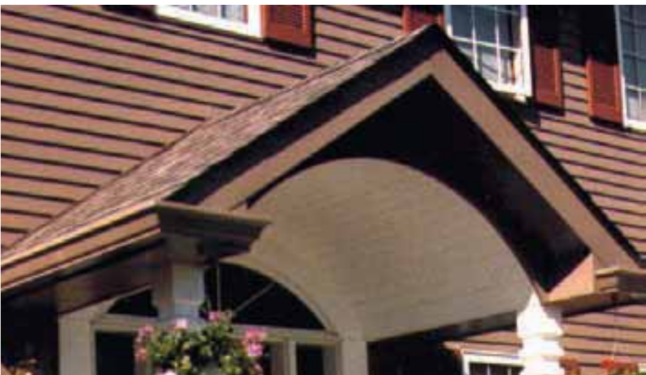
Above: Berridge Colonial Siding
