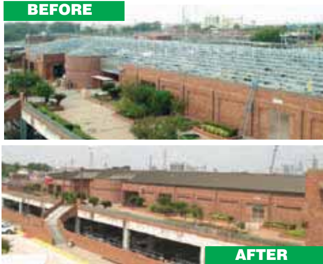
These photos illustrate how a Berridge "Vantage Point" retrofit roof system provides a totally new design appearance plus watertightness integrity.
