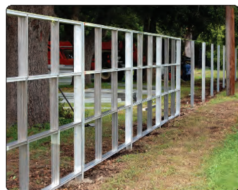
Fence structure made from 24 GA Spaceframe components & 16 GA C-Channel posts.
