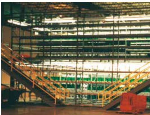
Multi-level Wide Span Pick Module
