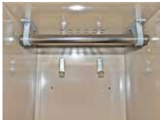
1" diameter coat rod and brackets fastened beneath ventilated shelf on garment side
