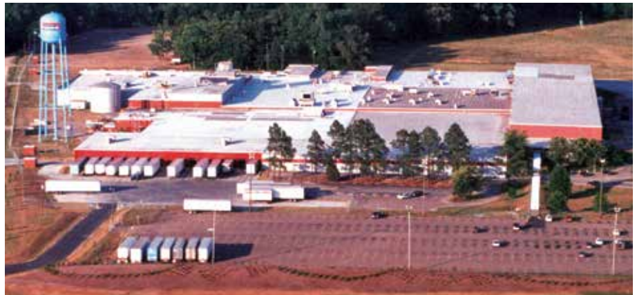
Manufacturing facility in Hamilton, NC
