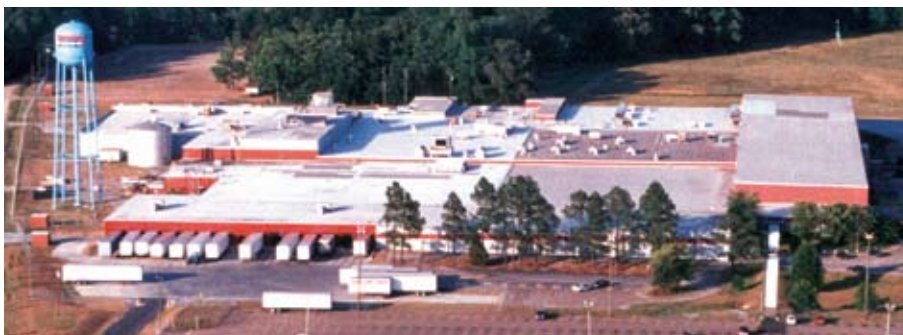
Manufacturing facility in Hamilton, NC
