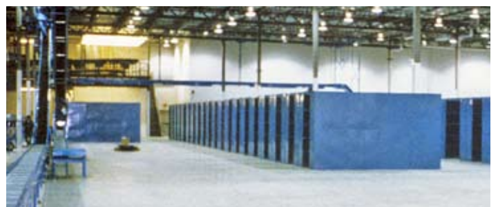
Distribution Warehouse for consumer goods producer.
