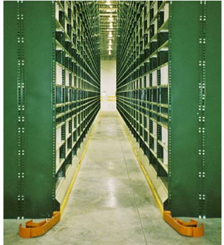
Truck parts distribution center with guide rail.
