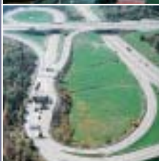
Pennsylvania Turnpike - Pennsylvania, USA
