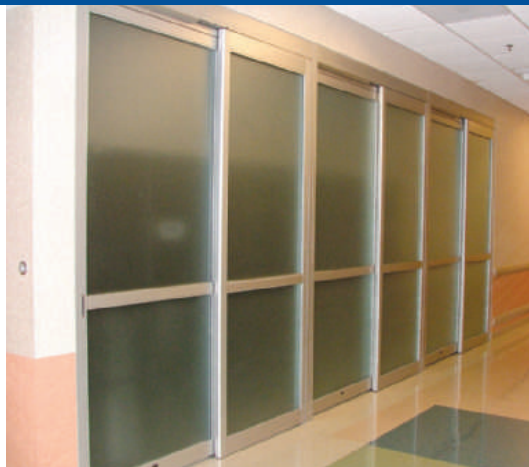
Corridor of 2-Panel ICU Packages
