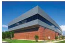
Page 26 South Texas Research Facility San Antonio, TX A: Rafael Vinoly Architects C: Vaughn Construction D: Wade Architectural Systems
