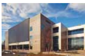
Page 22 Sherwood Middle School Shrewsbury, MA A: Lamoureaux Pagano Architects C: Gilbane Building Company D: LYMO Construction
