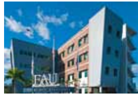
Page 23 Davie West Building Florida Atlantic University/University of Florida Davie, FL A: Schenkel Shultz C: Pirtle Construction Company D: Cladding Systems
