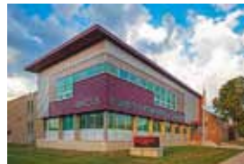
Page 25 Lincoln Elementary Louisville, KY A: Bravura Architects D: D T & Associates, Inc.
