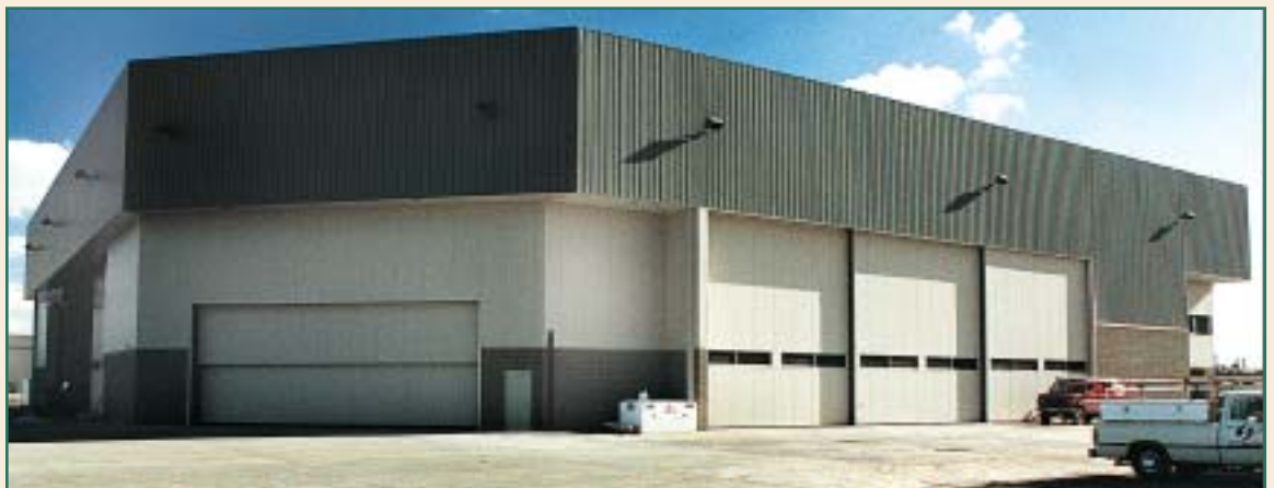
AMERICAN STORES' innovative corporate hangar in Salt Lake City was constructed by CONTINENTAL ENGINEERING CONSTRUCTION . This unique facility houses three different FLEMING SERIES 100 doors. On the near side (shown) is an 85'-0" wide by 28'-0" high 3-leaf Motor Operated UNIDIRECTIONAL door system. On the far side is a 100'-0" wide by 28'-0" high 4-leaf Motor Operated BIPARTING door system. In between the slide doors is a 40'-0" wide by 16'-0" high 2-section Motor Operated VERTICAL LIFT door.
