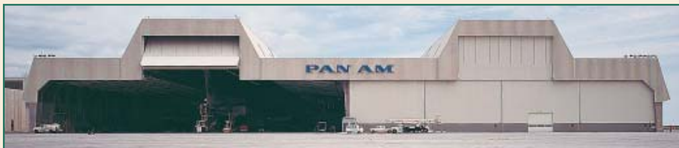
Built originally for PAN AMERICAN WORLD AIRWAYS at Kennedy International Airport, this hangar features four bays; each 265' wide and has 4 coupled Fleming Slide Doors controlled from cabs at each end of the "Train." Fleming CANOPY DOORS 80' wide by 35' high pass the high tails of B-747's. VERTICAL LIFT DOORS 21' wide by 16' high admit service vehicles.
