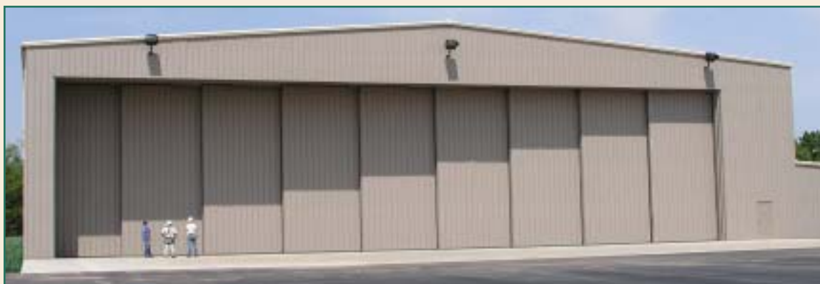
NISSAN'S new corporate hangar in Smyrna, Tennessee uses a 9-leaf Motor Operated SERIES 100 UNIDIRECTIONAL set of hangar doors in a 120'-0" wide by 28'-0" high opening.
