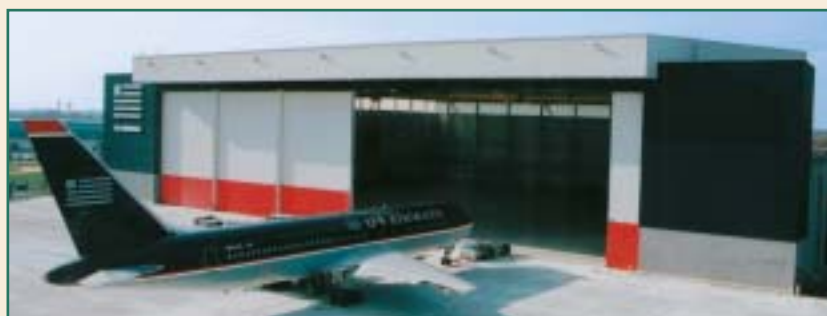
USAIRWAY'S colorful Line Maintenance Hangar at Philadelphia International Airport. This unique facility features a clear opening of 295'-0" wide by 66'-6" high and is filled by a 6-leaf INDIVIDUALLY MOTOR OPERATED Series 500 door system.
