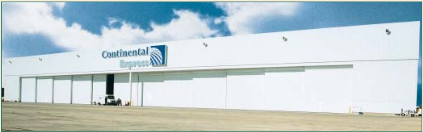
100 SERIES DOORS: To service its large fleet of Regional Jets, Continental Express at Knoxville, Tennessee uses a Fleming 12-leaf INDIVIDUALLY MOTOR OPERATED door system for a 360'-0" wide by 28'-0" high opening.
