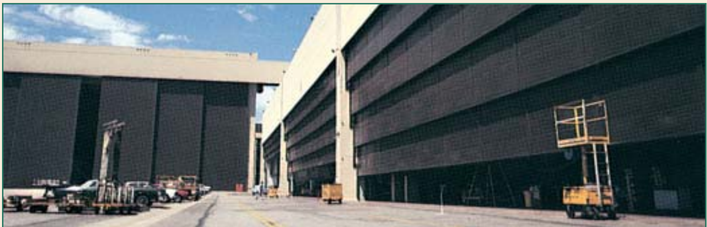
BOEING/McDONNELL DOUGLAS's Long Beach, California Facilities has three banks of 4-section motor operated VERTICAL LIFT doors 200'-0" wide by 45'-0" high. In the background is a sliding door system 350'-0" wide by 100'-0" high built for the Engineering Test and Evaluation Facility.
