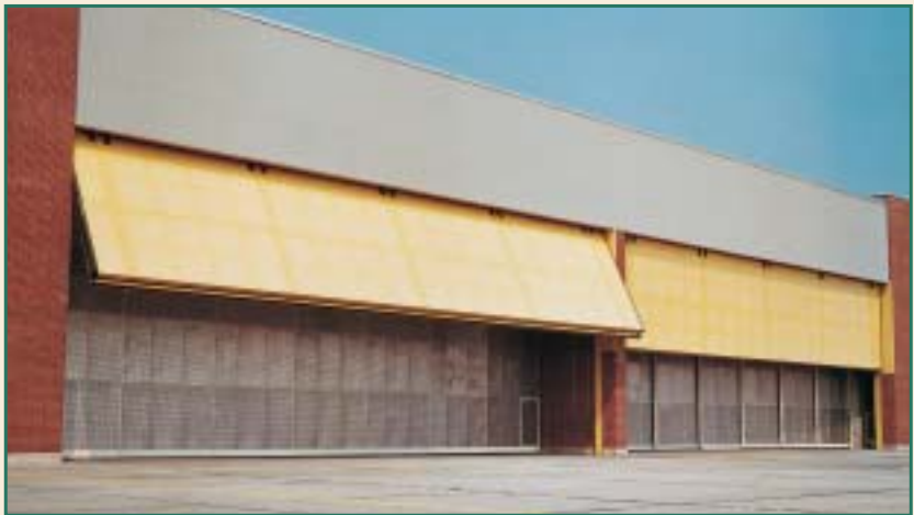
GRUMMAN Aircraft's Paint Building at Bethpage, Long Island, uses two 82'-0" wide by 27'-0" high Fleming Motorized TELESCOPIC CANOPY Doors with two sets of unusual Air Filter Sliding Doors behind them.
