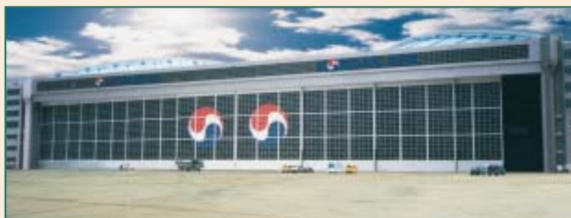
KOREAN AIR'S uniquely designed new Operation Center at Kimpo International Airport in Seoul, Korea houses an 8-leaf individually motor operated Fleming Series 500 door system for a 578'-0" wide by 83'-0" high clear opening. The doors are clad with a Lexan curtain wall system from 10'-0" A.F.F. elevation to within 4'-0" of the top and are designed for typhoon winds.
