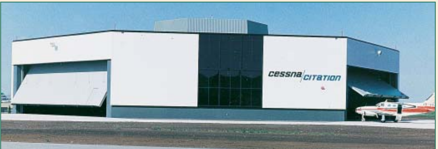
CESSNA'S CITATION Jet Facility in Wichita, Kansas, uses three Fleming Motorized UNBRACED CANOPY Doors 80'-0" wide by 21'-6" high.
