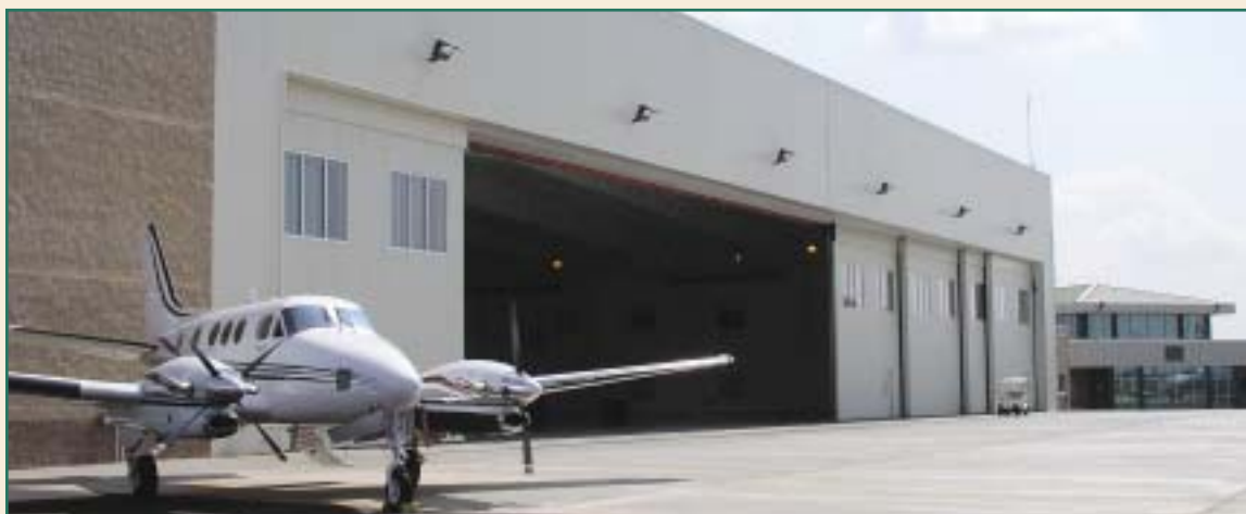
HAWKAIRE'S high tech. facility at Carlotte-Douglas International Airport was designed by Little & Associates. This innovative facility has two Fleming Series 100, 4-leaf FULL FLOATING GROUP hangar door systems in a 212'-0" wide x 27'-11" high clear opening.
