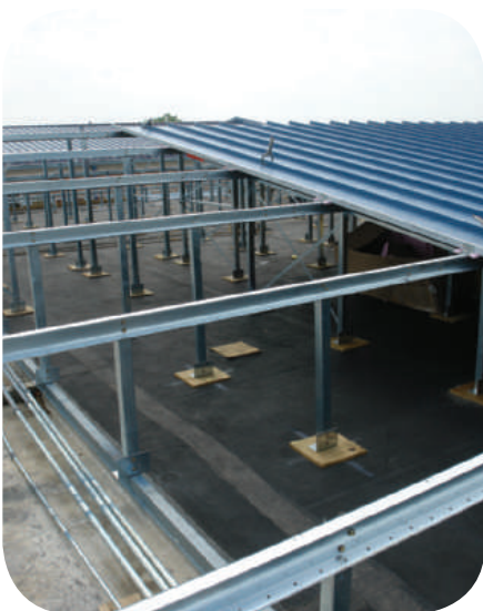
A Butler reroofing system is a long-term solution that saves the cost and inconvenience of tearing off an existing roof.
