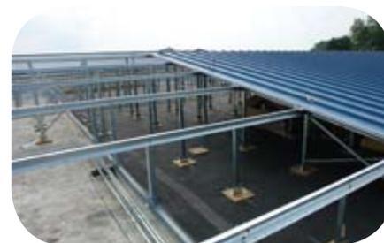
The slope build-up retrofit system, for complicated rooflines.
