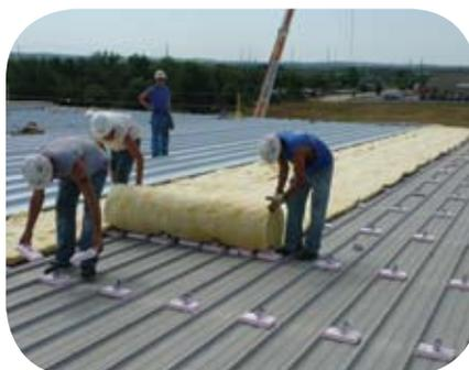
The MR-24 low-profile metal-over-metal retrofit system allows for a maximum 3" of blanket insulation.
