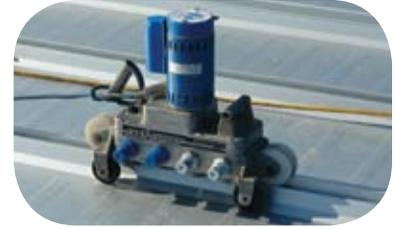
Butler's exclusive Roof Runner® completes the industry's only field-formed 360-degree Pittsburgh double-lock seam.
