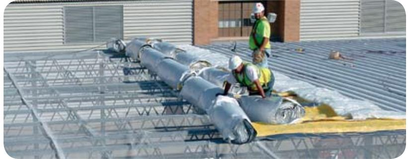
An alternate fall protection and insulation support system, Sky-Web®, is also available.
