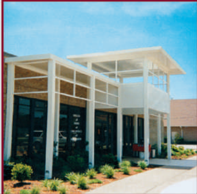
Entrance Canopy Tyler, TX
