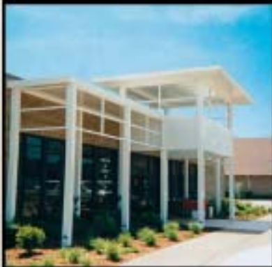
Entrance Canopy Tyler, TX
