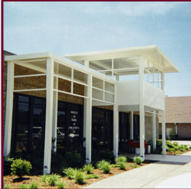
Entrance Canopy Tyler, TX
