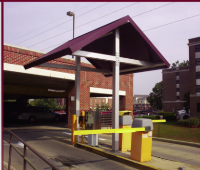
Ticket Booth Cover Tuscaloosa, AL
