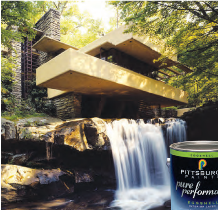
PPG Pure Performance Coatings were used in the restoration of Frank Lloyd Wright's Fallingwater in 2001.
