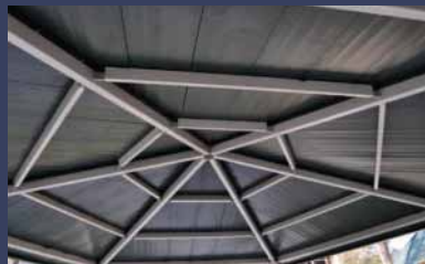
18" wide standing seam panel • galvalume steel, ASTM A792 Gr 50
