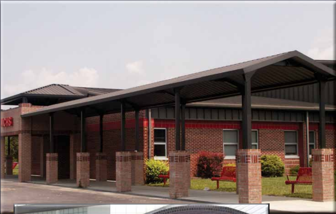
Illini walkway, custom brickwork
