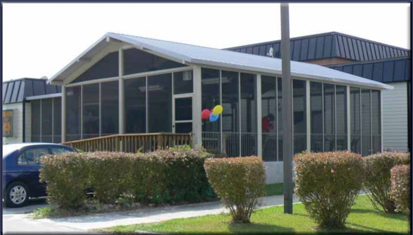
Illini, with wall system
