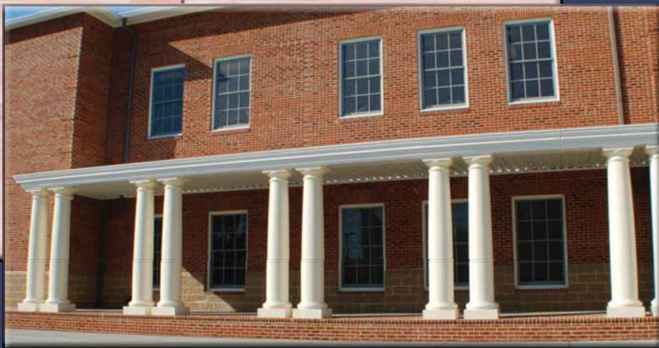
Algonquin Walkway with Custom Trim & Columns
