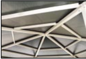
Insulated sandwich panel 3" thick x 48" wide, high density polystyrene between two layers of white stucco embossed .032 aluminum.
