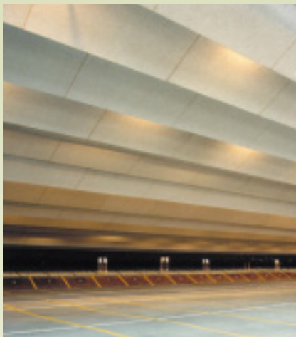
▲ Tectum panels used for sound control in the Los Angeles, CA, Police Department Firing Range.
