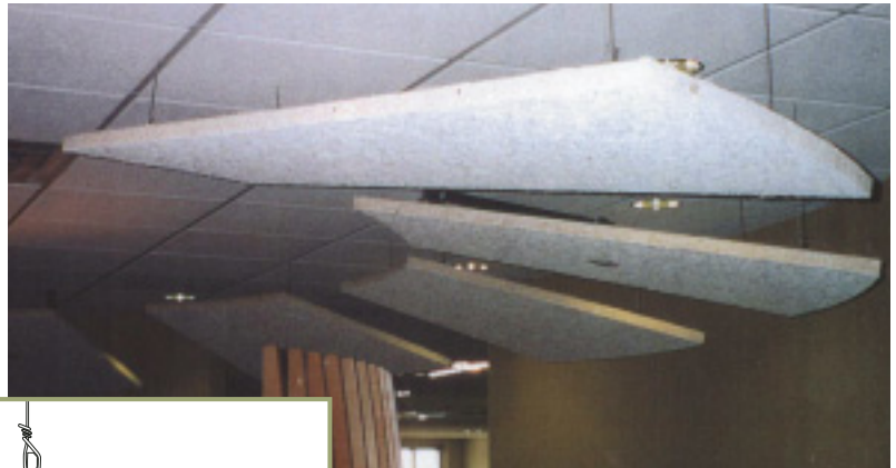
▲ Tectum Cloud Panel Installation
