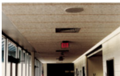
▲ Full-Span Corridor Panels- Royal Middle School, TX
