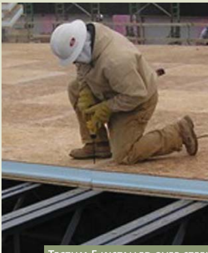
TECTUM E INSTALLED OVER STEEL.
