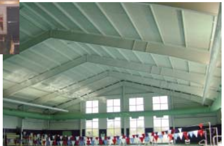
Lorain Co. Metro Park Pool (Lorain, OH) ▼ Tectum III Roof Deck
