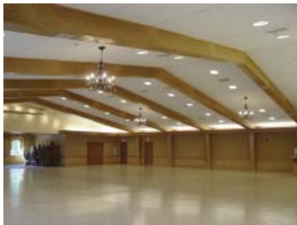
◀ Bay District Volunteer Fire Station (Lexington Park, MD) Tectum I Roof Plank
