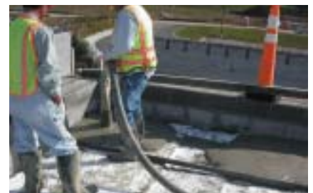
▲ Installation of lightweight insulating concrete over a Tectum I roof deck.
