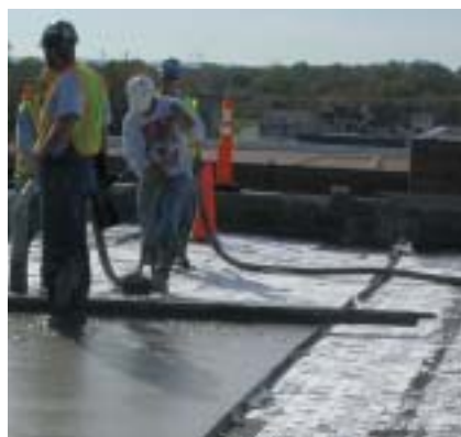
▲ Installation of lightweight insulating concrete over a Tectum I roof deck.
