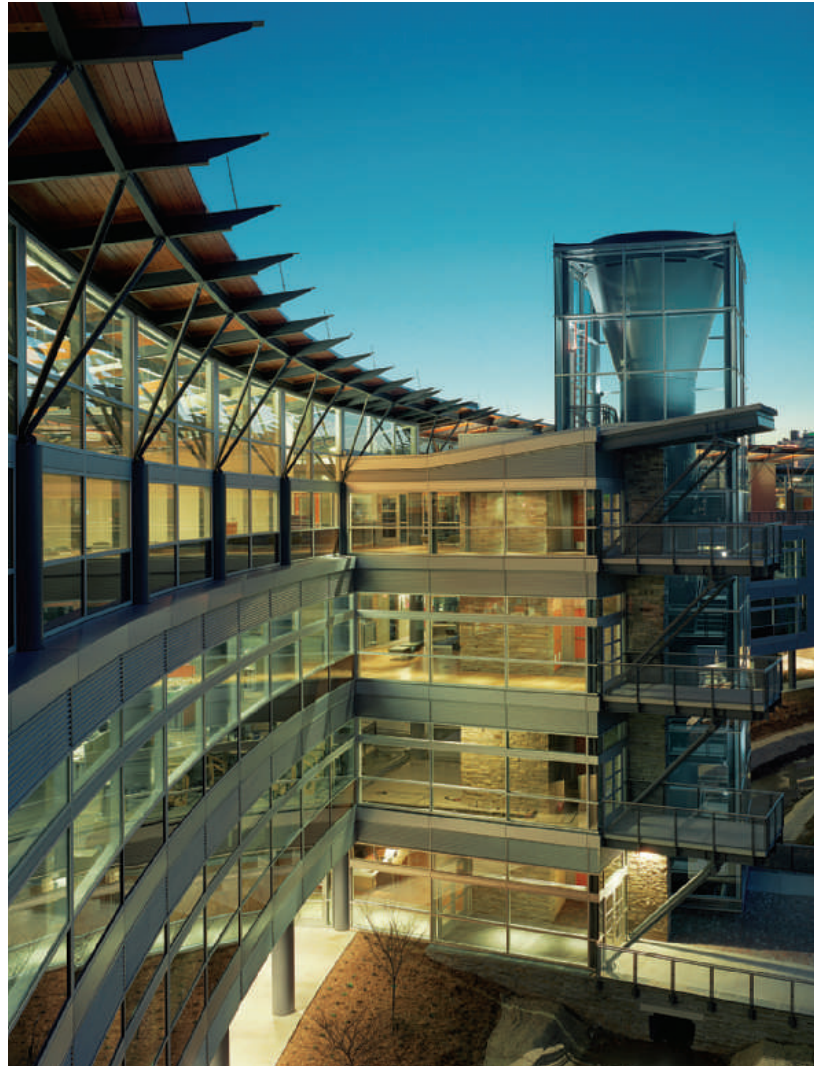
Top Photo: Georgia Highlands College - Cartersville, GA Architect: Cooper Carry Architects General Contractor: Aviation Construction Inc. Roofing Contractor: Atlanta Metal Systems LLC Material: TCS II Profile: Snap-Clad, gutters & downspouts
