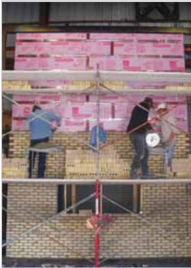
NFPA 285 test wall under construction.
