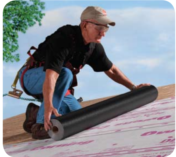
Figure 1: Typical Underlayment Installation
