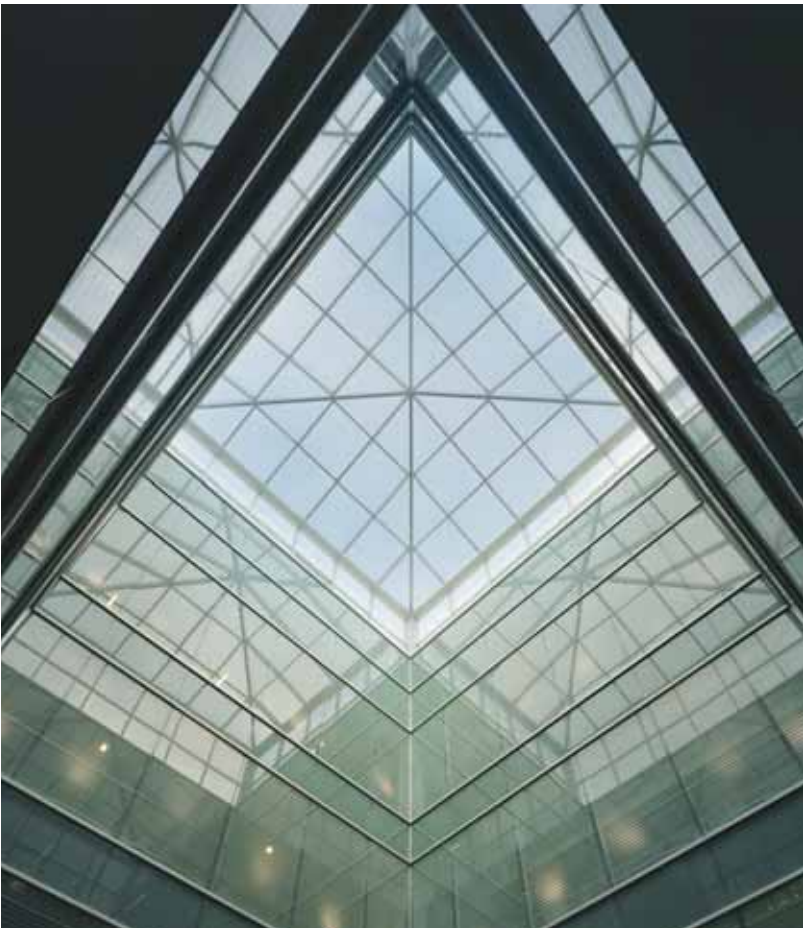
THE CENTER FOR THE INTREPID-BROOKE ARMY MEDICAL CENTER Fort Sam Houston, Texas Architect: Smith Group
