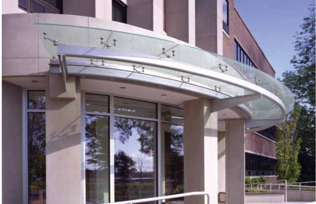
NATIONAL STARCH AND CHEMICAL CORPORATION Bridgewater, New Jersey Architect: Henderson Design Group
