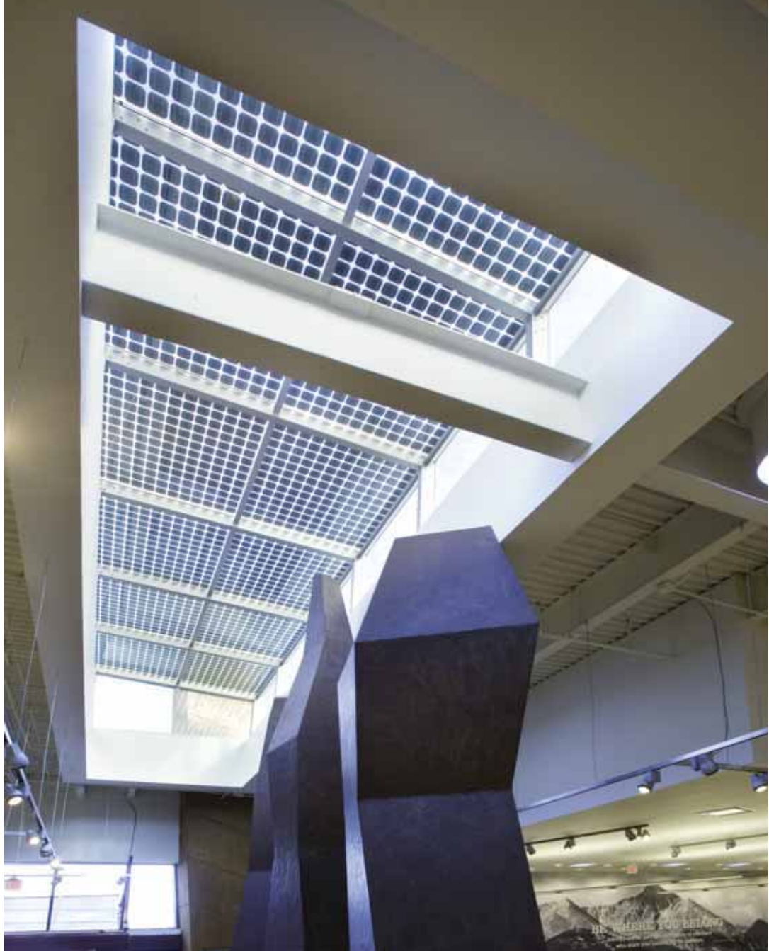
REI RETAIL STORE Boulder, Colorado
