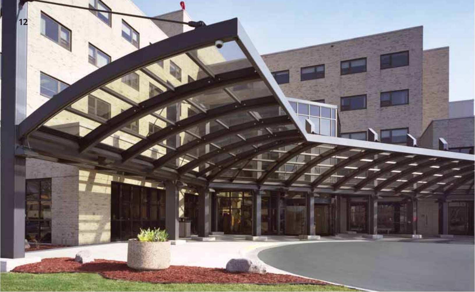
ST. MARY'S HOSPITAL EMERGENCY DEPARTMENT
