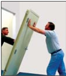
Set preassembled doorway in opening.
