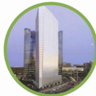
Tour Granite, France
