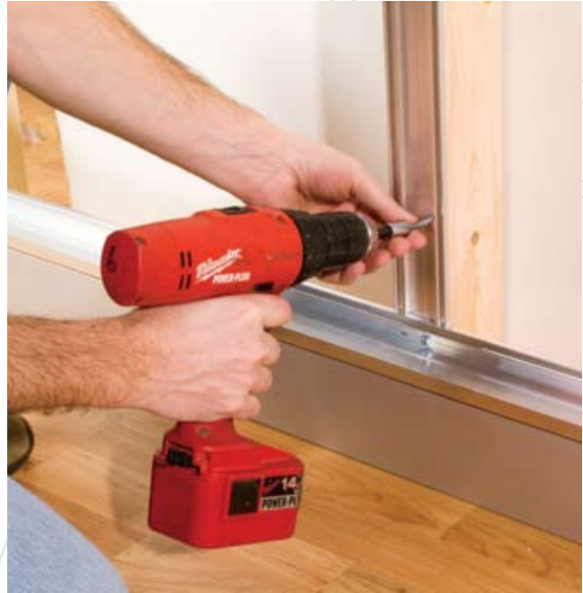
Proprietary wall rail hardware that holds panel assemblies is easily installed with simple tools
