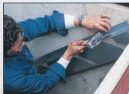
Nail steel Stair Stringers to areaway sidewalls.
