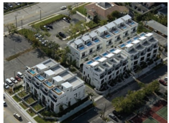
19 Rooftop Endless Pools Pompano Beach, Florida
