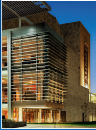
Horizontal Sunshades University of California Davis Performing Arts Center; BOORA Architects, Inc.
