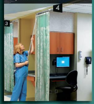
**Step 2** Load a clean curtain onto the carrier. Using the Qwik Switch wand, push the track back up to the ceiling, and the Qwik Switch locking unit will lock the track back into position.
