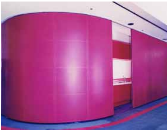
San Diego Convention Center: Manually operated panels create a security screen. Panels have perforated-steel, sound absorptive faces and paint finish.
