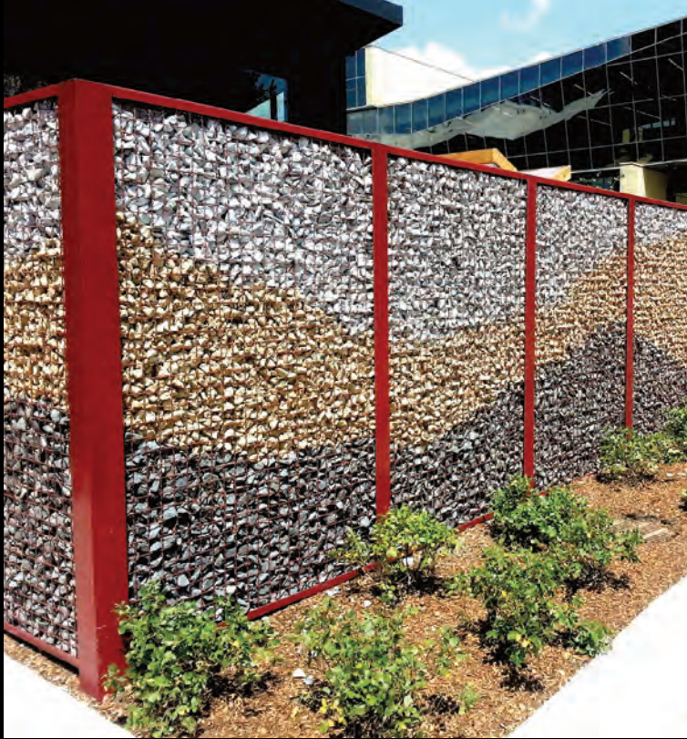
McNICHOLS ECO-ROCK™ was fabricated into a fence and filled with rocks of various colors.
