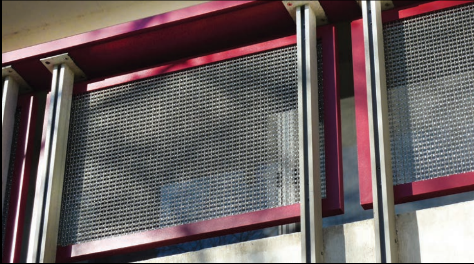
McNICHOLS Techna™ 3156 in 316 Stainless Steel was specified for infill panels of the balconies of this Providence, RI housing.
