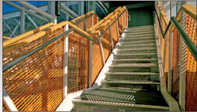
Bar Grating infill panels were powder coated with a customer specified color providing a safe and secure corridor between building complexes.
