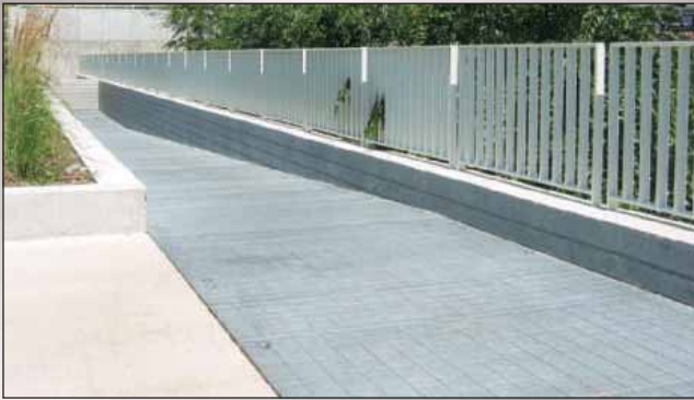
Hot dip galvanized panels of Bar Grating were easily fabricated on-site for this walkway providing for a maintenance free, long service life.
