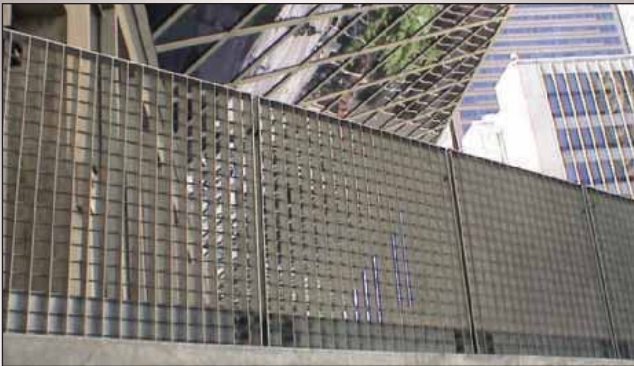
Panels of Bar Grating were used in the design and construction of this barrier. Securely anchored, they provide security, ventilation and visibility.
