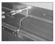
**Step 3.** Squeeze bellows, apply flange to snap line and nail 8" oc starting 1" from end with fasteners appropriate for wall material
