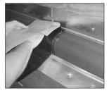
Step 6. Install 6" wide peel & stick splice tab, removing backer sheet ahead of application. Extend tab onto roof 4" beyond metal flange. On wall flange trim tab at top of flange
