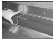
**Step 3.** Squeeze bellows, apply flange to snap line and nail 8" oc starting 1" from end with fasteners appropriate for wall material
