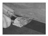
**Step 1.** Snap line 4" both sides of joint opening & trowel mastic compatible with membrane to line, both sides
