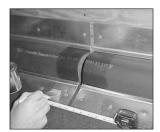
**Step 4.** Prime metal & bellows using brush 3" either side of splice and allow to dry tack free
