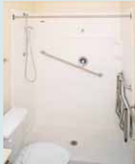
ADA shower floors, walls, seat, grab bar – Fulton, Missouri
