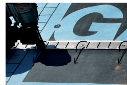
Install Battens & Hangers
