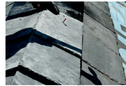
Install Ridge Vent, Trim Slates, And Top Row Of Field Slates
