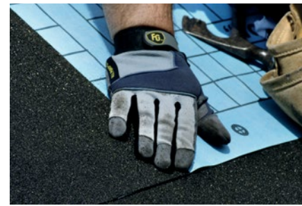
Apply Leak Barrier And Roof Deck Protection
