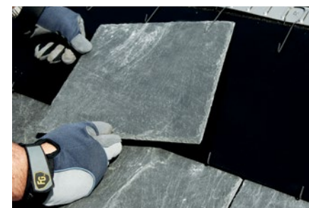
Insert UV & Moisture Barrier And Field Slates
