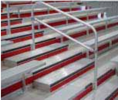
Code compliant markers with no external fasteners
