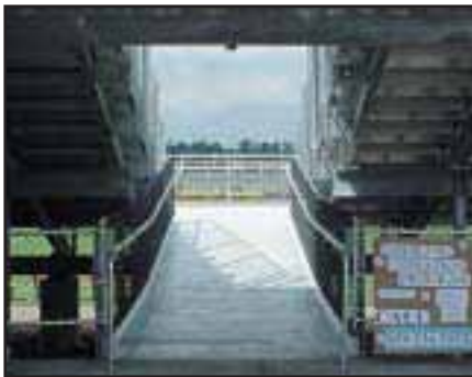
Vomitory exit with ramp to grade.
