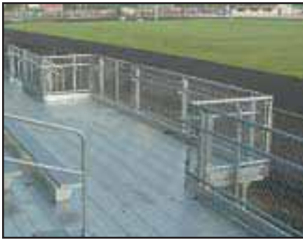
Front walkway with handicap platform extension.
