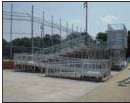
Handicap ramp with landings to main bleachers.
