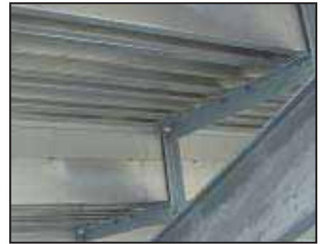
Galvanized steel understructure with welded aluminum decking.
