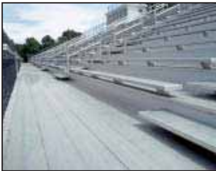
Welded deck walkway and decking.
