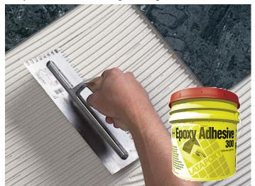
to embed tile and adjust level. Check mortar for complete coverage by periodically removing a tile and inspecting bedding mortar transfer onto back of tile.
