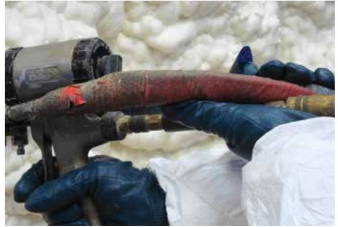
Consideration needs to be given to the potential for condensation. It is important that adequate thicknesses be applied to reduce the possibility of condensation on the warm and humid surface side of the insulation. When applying SPF in structures or climates where moisture is an issue, it may be necessary to include an additional vapor retarder/barrier.
