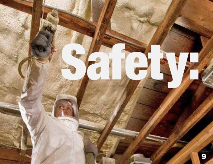
This section introduces the importance of safe handling of materials and the use of required personal protective equipment (PPE) when applying SPF.
