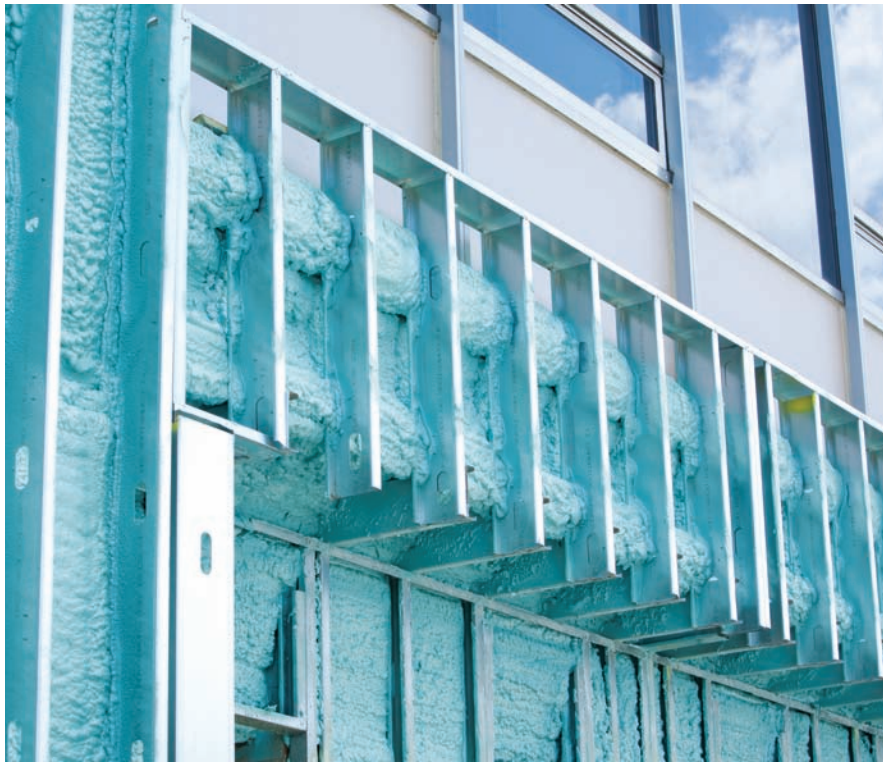
In the photo above, SPF has been applied under a cantilevered wall section.
