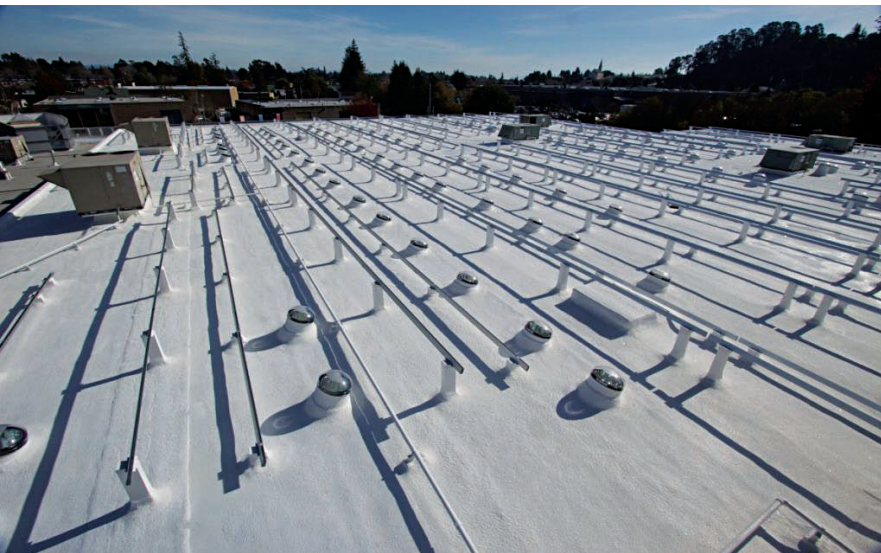
A spray-applied polyurethane foam (SPF) roof, prepared for photovoltaic (PV) cells. Photo © Central Coating Co. Photo courtesy Bayer MaterialScience LLC
