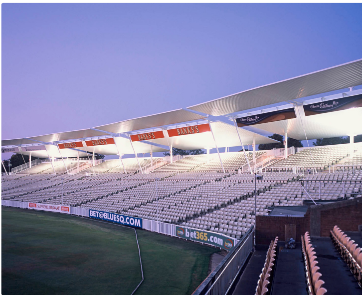
The Vega TM illuminates a stadium ceiling producing amazing indirect light.
