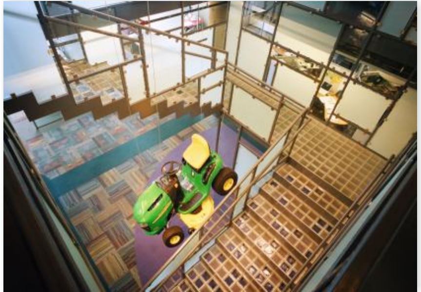
STEEL FRAMED STAIRCASE WITH INLAID GLASS BLOCK.
