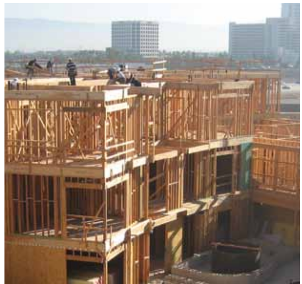
To accommodate potential shrinkage, engineers must allow for adequate movement between the structural elements and building finishes such as masonry veneer.
