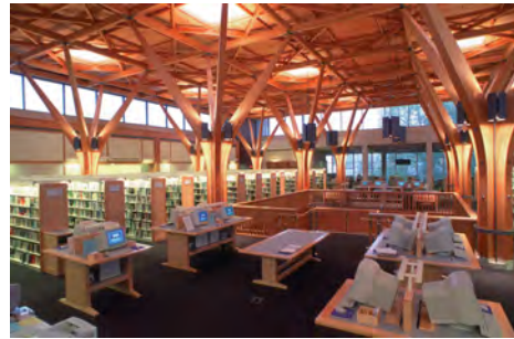
Figure 10: Type IV Construction
