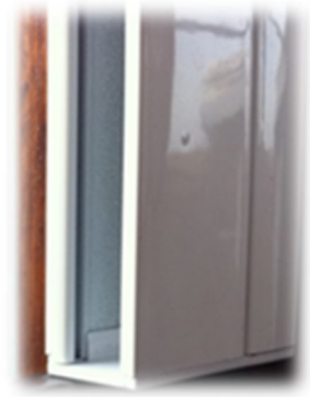
Close up of side channel of roller blind.
