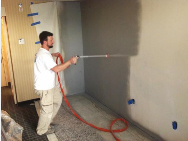
Spraying first base coat
