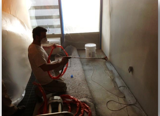
Spraying first base coat
