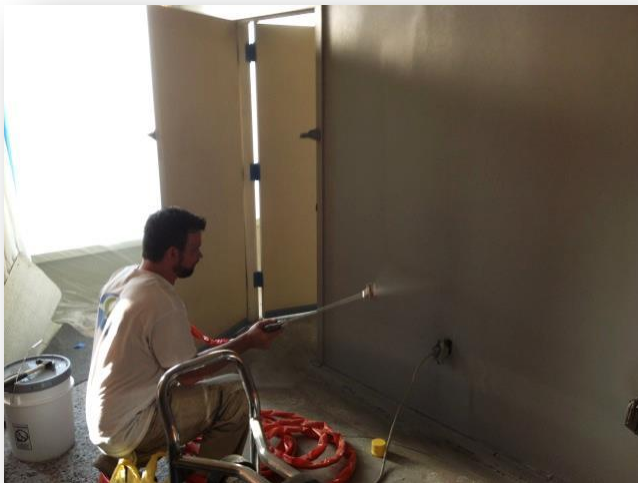
Spraying second base coat
