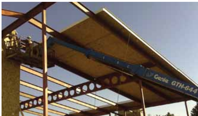
Fox Construction (above)- installed 12 Jumbo panels per hour.
