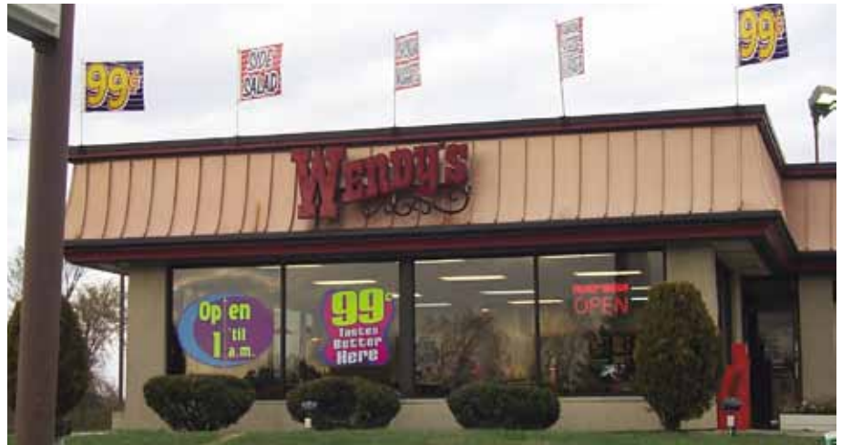
FAST FOOD - FAST CONSTRUCTION - 28 DAYS BY ROCKFORD CONSTRUCTION
