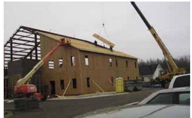
Large panel rigged at roof angle, when lifted.
