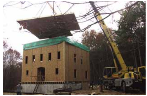
Large panels, assembled on the ground, then lifted.
