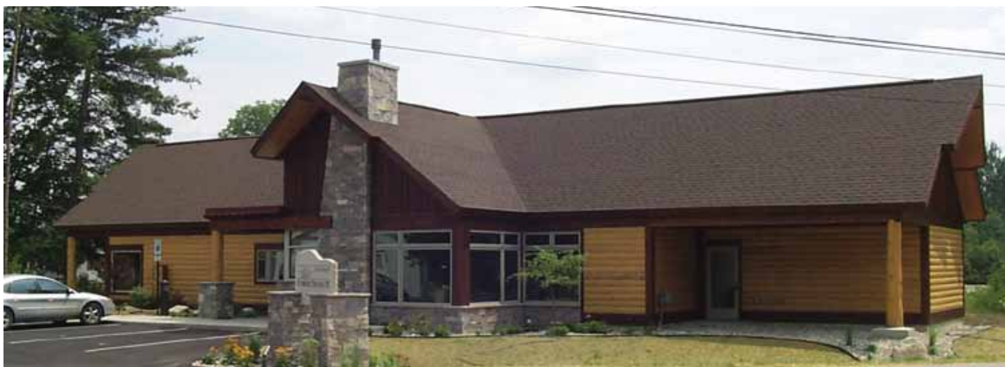
Half-log siding applied over SIPs
