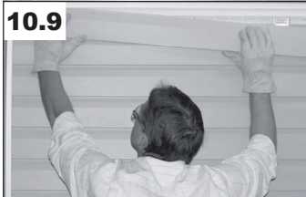
10.9 Slide crimped side of top panel up and lock into FAST-FINISH™ trim adaptor.
