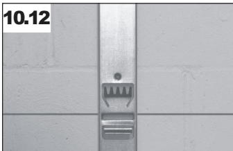
10.12 Align chalk line with top of the finger slot on the SIDING-MASTER™ strip and draw chalk line as in section 1.0.
